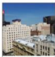
Aegis Building Marsh...
