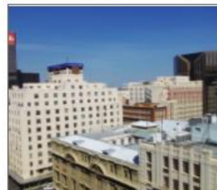
Aegis Building Marsh...
