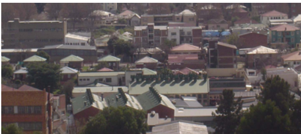
Figure 20 : The roofscape of the Lorentzville Industrial Zone between Victoria and Frere Roads
