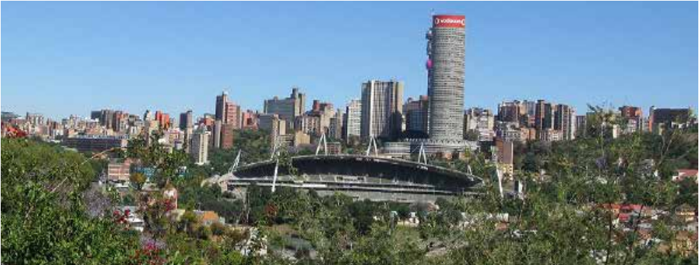
Figure 21 : View across the Ellis Park Sports Precinct from the East
