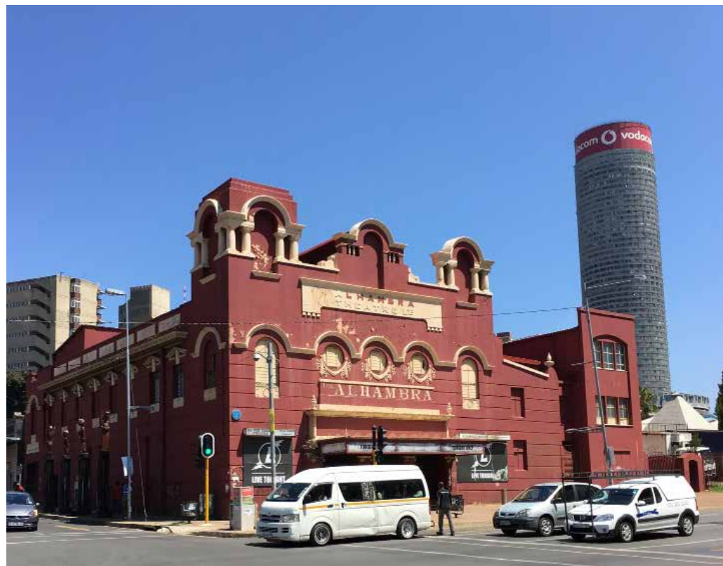
Figure 36 : Alhambra Theatre, one of the buildings of heritage significance located in New Doornfontein (Source: Johannesburg 1912 - Suburb by suburb research; https://johannesburg1912.wordpress.com )
